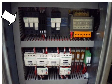
Fig. 6.10 – Accessibility to fuses
